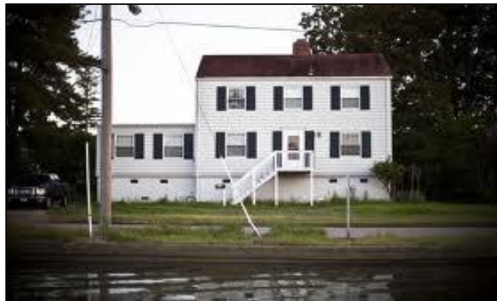
Fig. 8. Flooding in the Lafayette River area.
