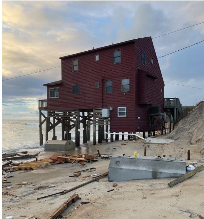
Figure 3: Debris Associated with House Collapse , NAT'L PARK SERV. (Sept. 20. 2024), https://www.flickr.com/photos/capehatterasnps/54008888865/in/album-72177720320480249 (showing three exposed, detached septic tanks plus debris at 23001 GA Kohler).
