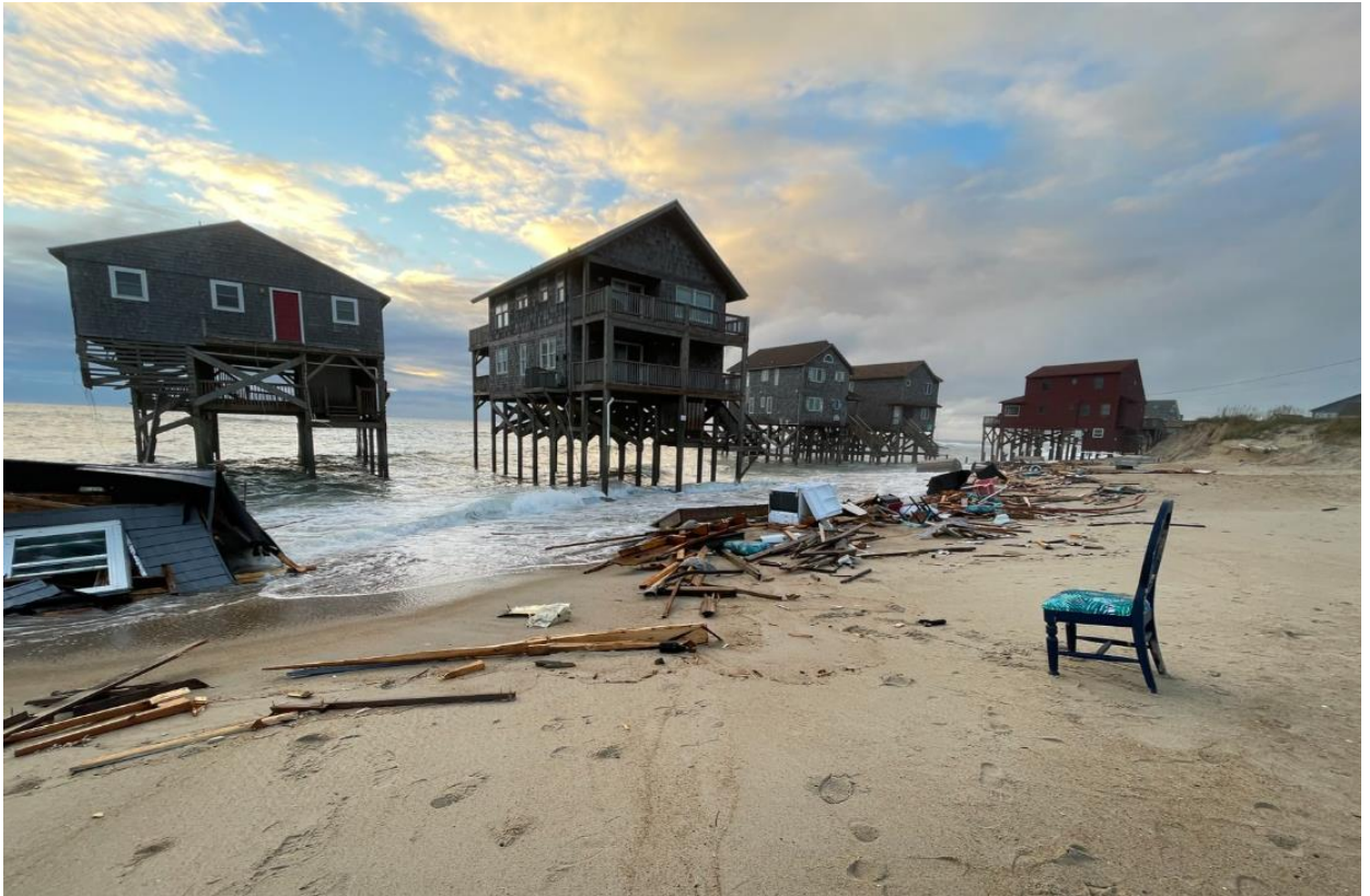
Figure 1: Debris associated with house collapse , NAT'L PARK SERV. (Sept. 20, 2024), https://www.flickr.com/photos/capehatterasnps/54008888455/in/album-72177720320480249 (depicting 23001 GA Kohler Court).
