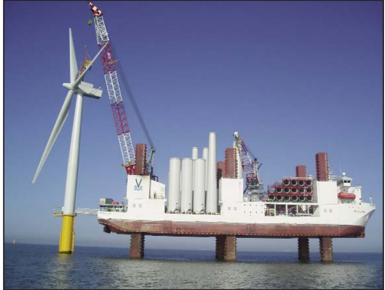
Photograph of wind turbine being erected courtesy of Centrica, PLC.
