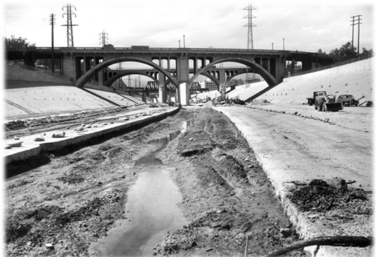
Photograph of Los Angeles River during construction courtesy of The National Archives.
