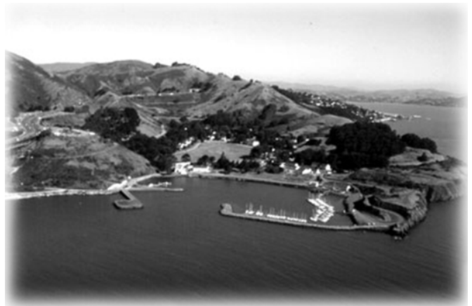
Photograph of Fort Baker courtesy of the National Park Service.
